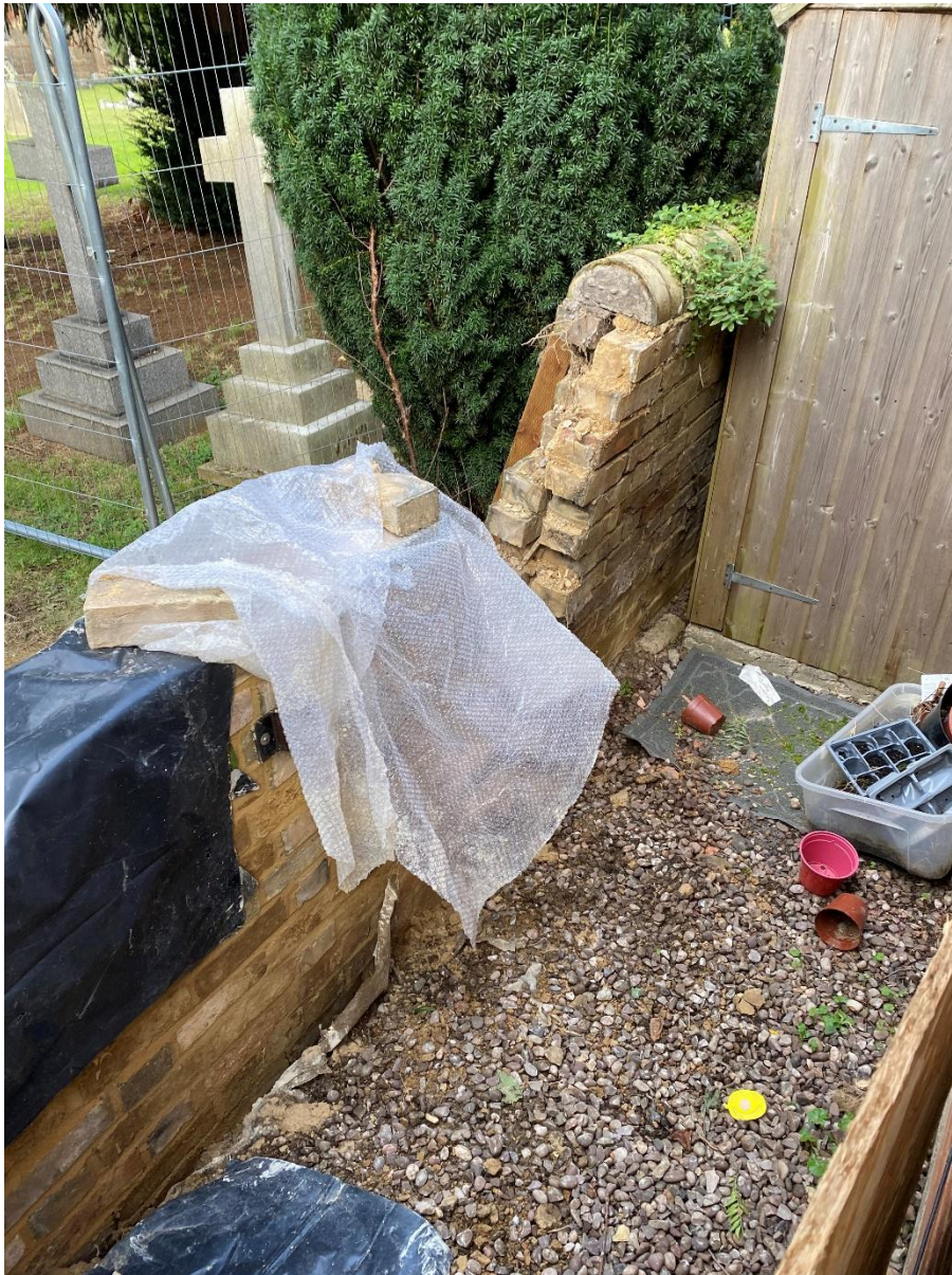
Appendix A: Picture of defective boundary wall.
