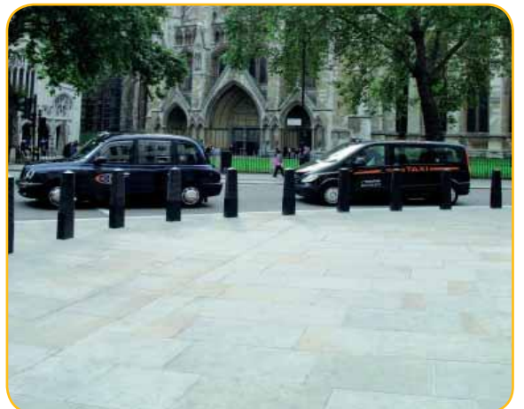
Marshall's Scoutmoor York Stone (diamond sawn) for pedestrian only feature areas
