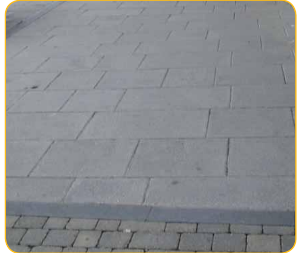
Marshall's Natural Saxon 450 x 600mm rectangular slabs
